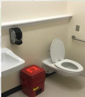
New restroom WMS nurses office
