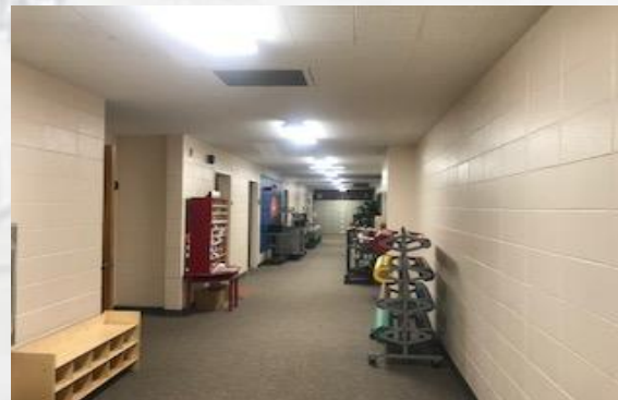
New LED lights Yale entry and main hallway.
