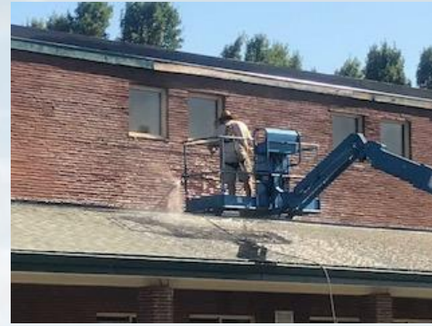
All brick work at WMS power washed and inspected.
