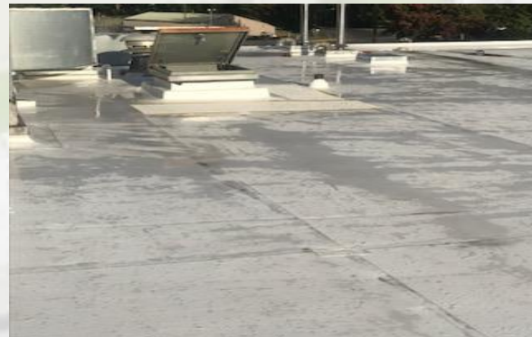
New TPO roof Green Gym
