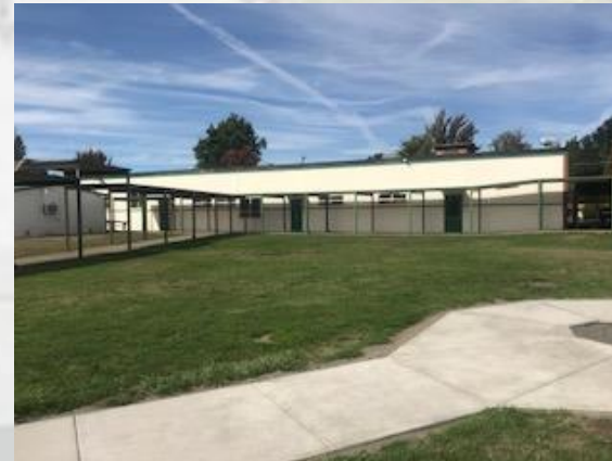
Building A,B,C repaint (building A shown)
