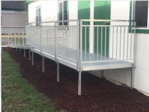
New ADA ramps installed at 3 locations.
